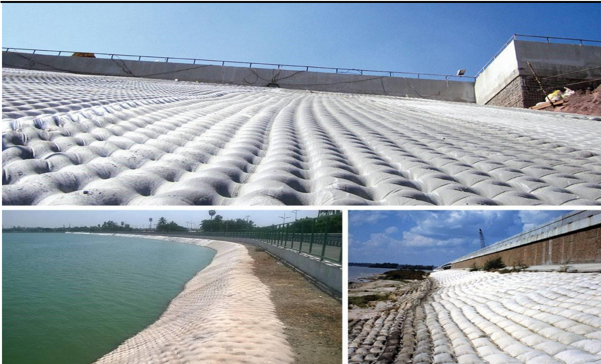
Fig. 1. Installed Tech-Revetment System
