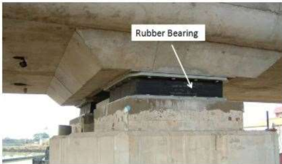
Fig :-5.3 Bearing in Bridge
