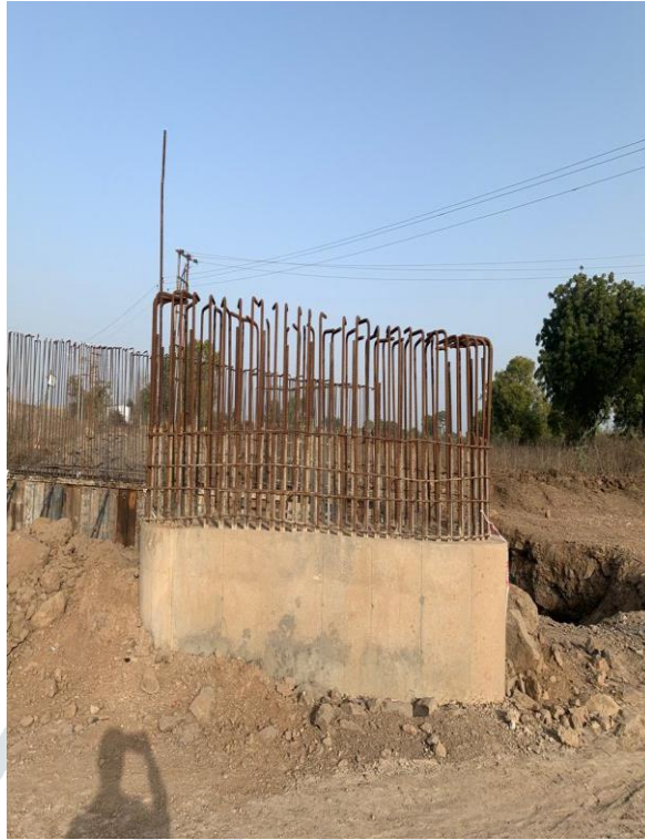
Figure 1.1: Partially completed column structure of NH-6
