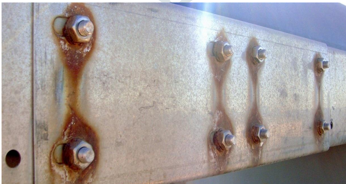
Figure 1.3: Galvanic corrosion
