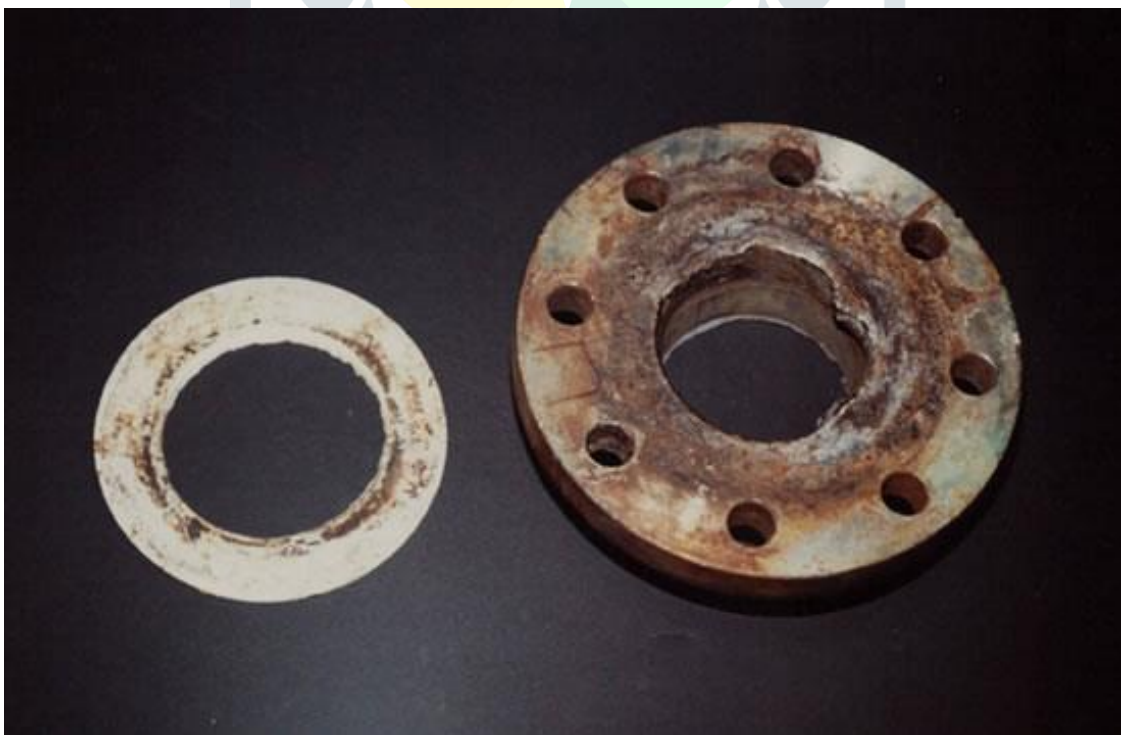
Figure 1.4: Crevice corrosion on a stainless steel flange
