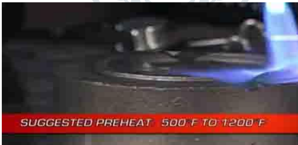
Fig 2.2 Cast Iron Welding Repair Preheating
