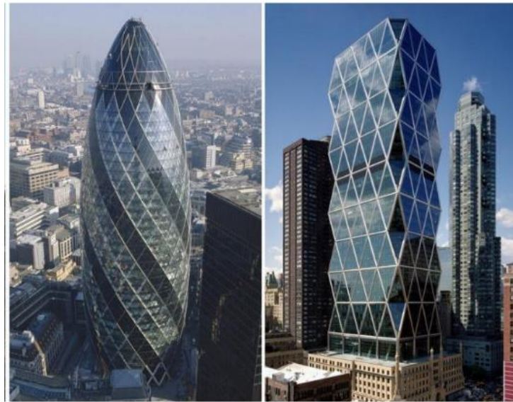
Figure 1. Diagrid buildings (a) Swiss Re in London (b) Hearst Tower in New York
