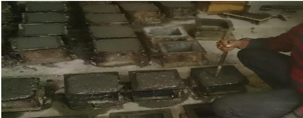
Fig: 1.4 Compaction by Hand
