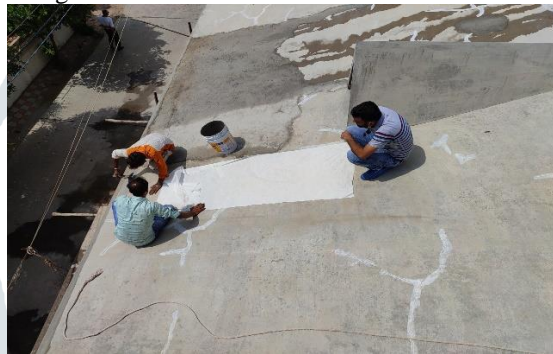
Fig 3.2. Membrane Type Waterproofing
