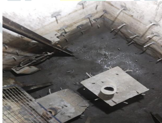
Fig 3.3. Injection grouting
