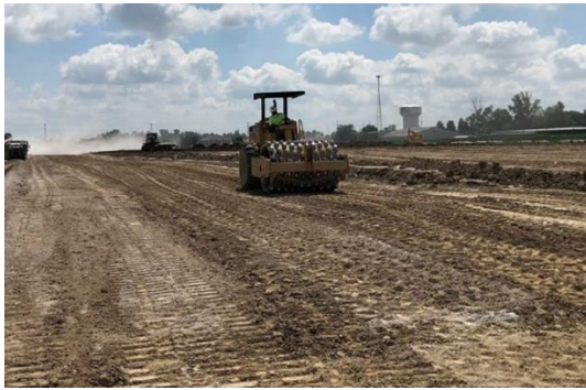
Figure No.1 Soil Stabilization
