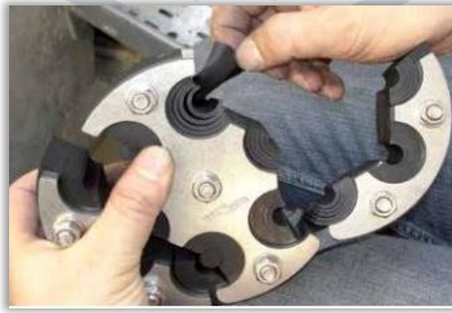
Figure 9: Split type multi-cable sleeve with rubber layers and cables passing
