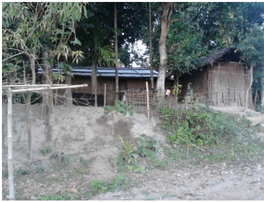
Plate 1: A Typical Assamese house with raised plinth
