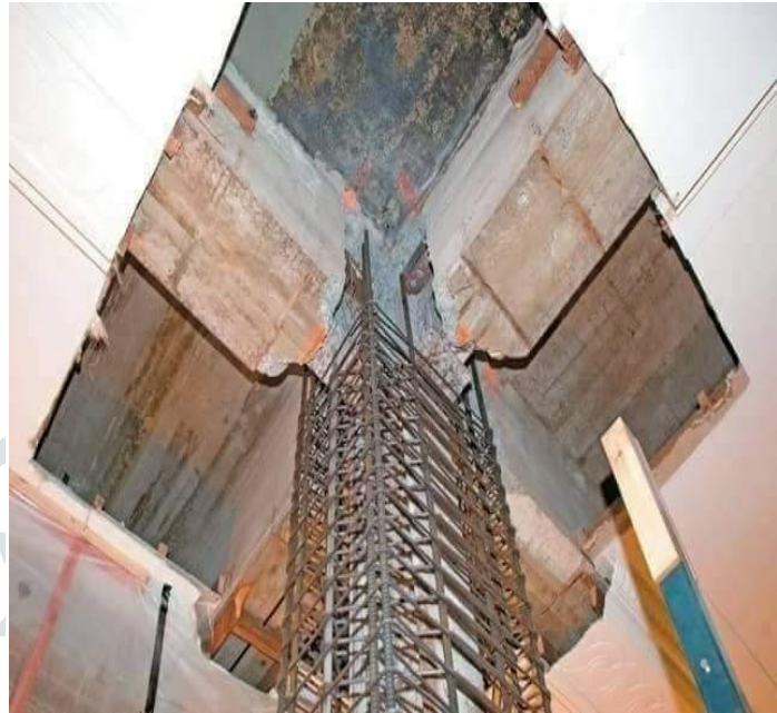
Figure 1.6 Jacketing on existing structure
