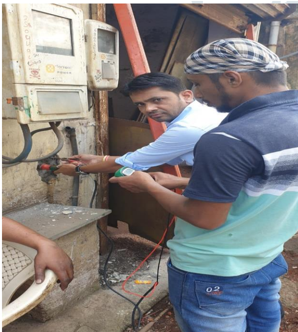
Figure 1.3 Half Cell Potential Test
