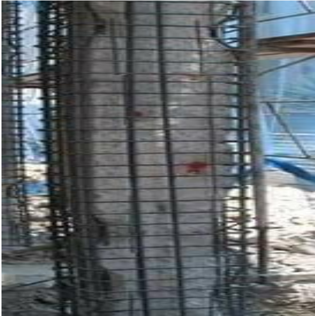
Figure 1.5 Jacketing on existing column
