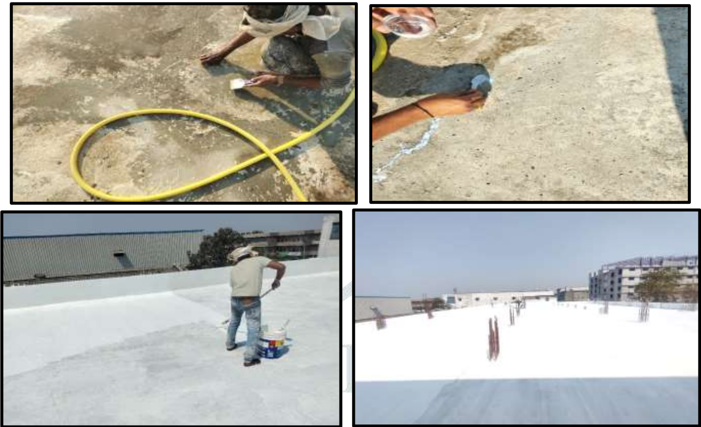
FIGURE 5.3 SITE OF TERRACE WATERPROOFING
