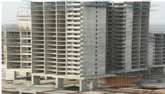
Figure 1:- Transfer slab With Shear wall
