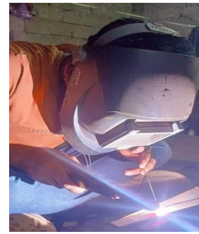
Fig. 3: Performing TIG Welding
