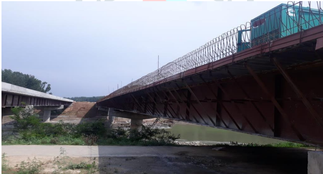
Figure 1- Construction of Bridge in Sangam by Ramky Infrastructure.
