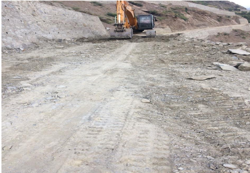
Figure 2- Road construction in Bankote, Banihal J&amp;K by Jehlum Construction Company
