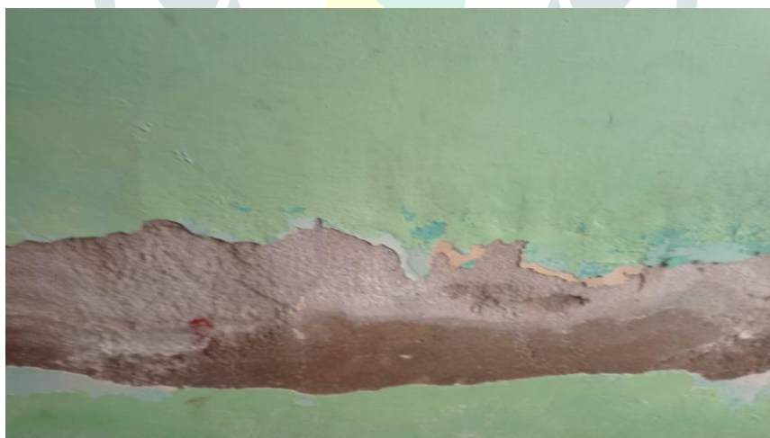
Fig.3 Fracturing due to creep
