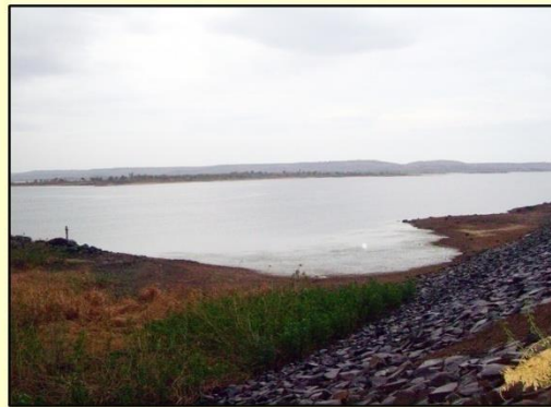
View of Siddheshwar Reservoir from Embankment
