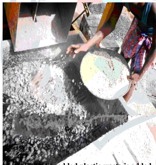
Fig 2: Shredded plastic waste is added
