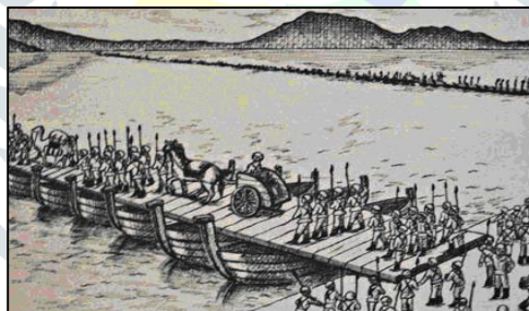
Fig. 1: Old Floating Bridge
