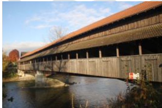
Fig. 3- Overview of Sins Bridge
