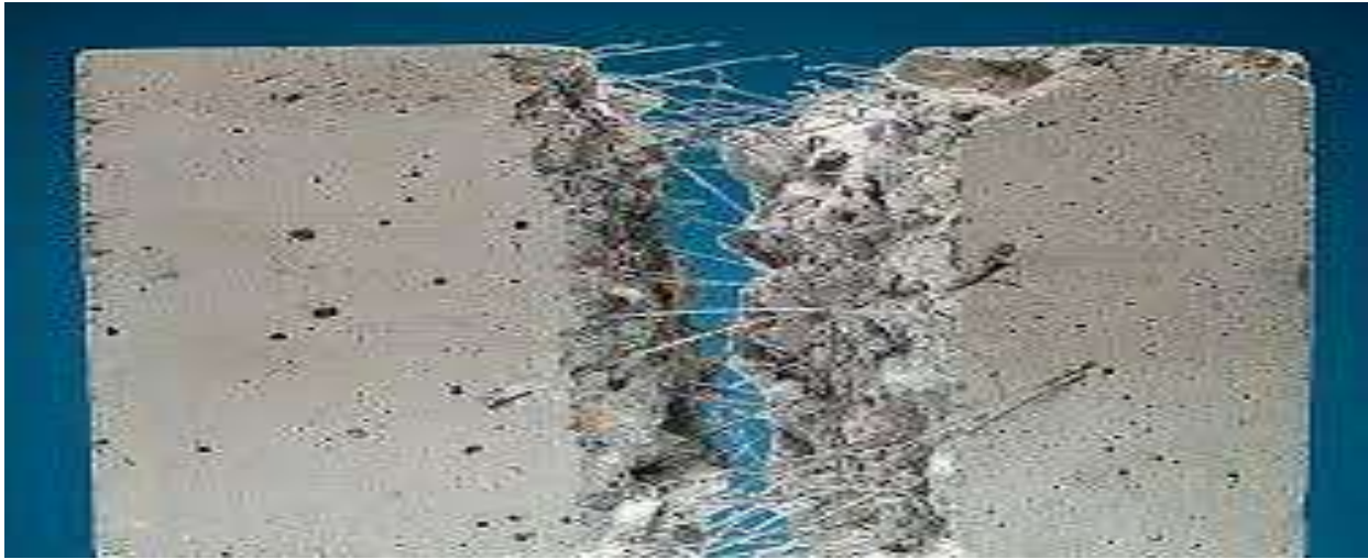
Fig. 1 Example of an image of fiber reinforced concrete.
