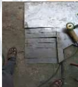
Fig 6:Cutting of theSheet Metal
