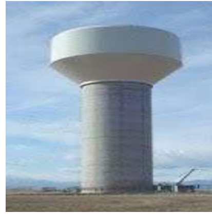
Fig. 3 Intze tank with shaft type staging
