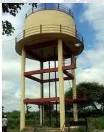
Fig. 1 Elevated R.C.C. Water Tanks
