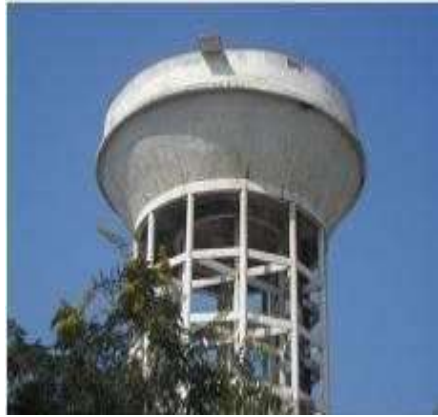
Fig. 2 Intze tank with frame type staging
