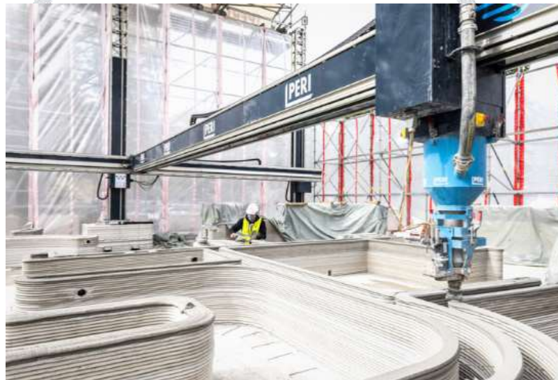
Figure 4: Illustrates the 3D construction process [ARCHDAILY].
