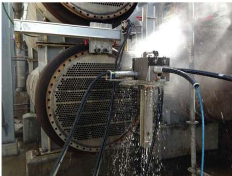
Figure 4: Illustrates the process of automatic cleaning used to clean heat exchanger with the help of water jets.
