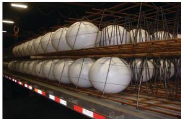
Fig. 2: Plastic Spheres Along With Reinforcement
