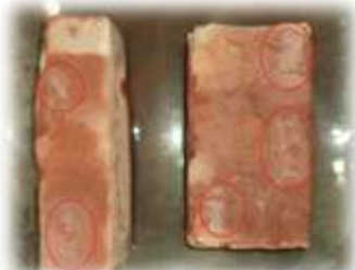
Fig.8: Photograph Showing Selected Pair of Second Class Brick with ‘Moderate’ Efflorescence on Red Marked Areas.
