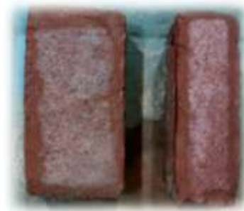
Fig.9: Photograph Showing Selected Pair of Third Class Brick with 'Heavy' Efflorescence.
