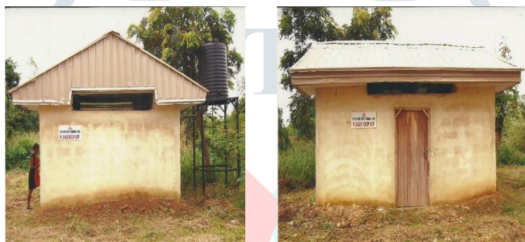
Fig. 2: Side and Front view of the completed evaporative cooler
