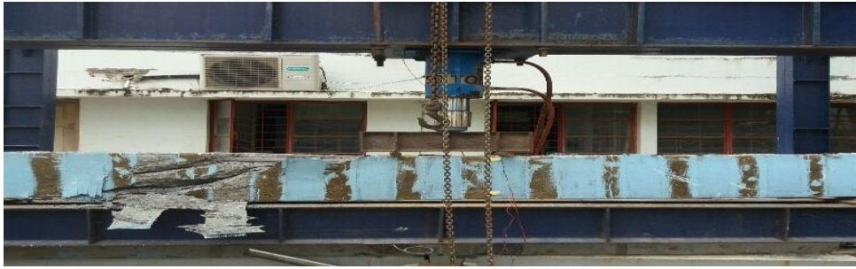
Fig.11.Failure mode of U-wrap strip beam-2
