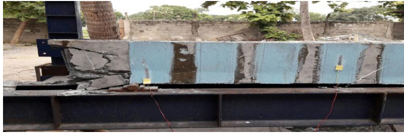
Fig.7 Failure Mode Of Side Strip Beam-2
