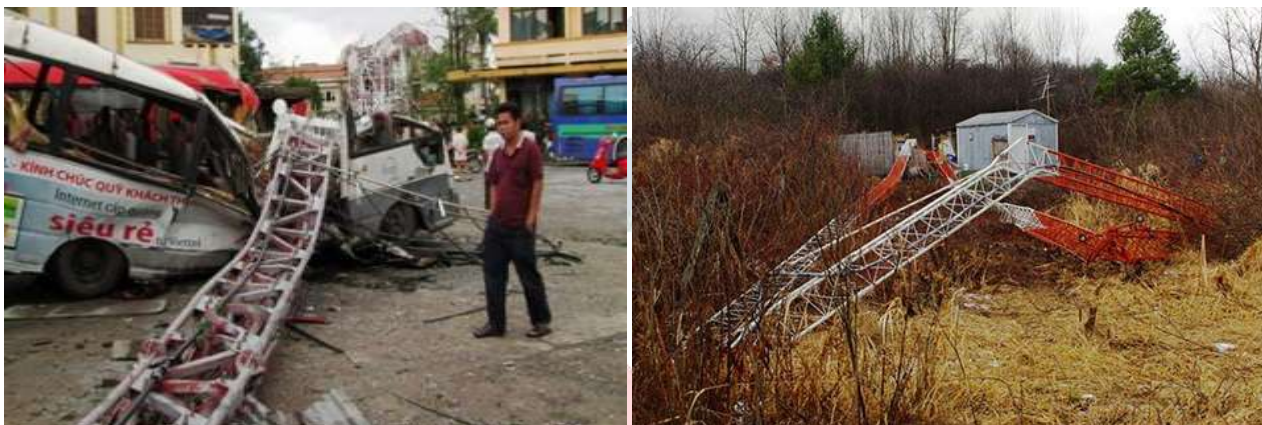
Fig. 1 Failure of guyed tower
