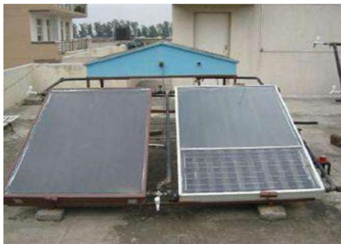
**Fig.11** Singh's hybrid single basin DS solar still integrated with PV collectors
