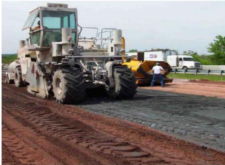
(Road Re claimer mixes Soil with Moist conditioned Fly Ash)
