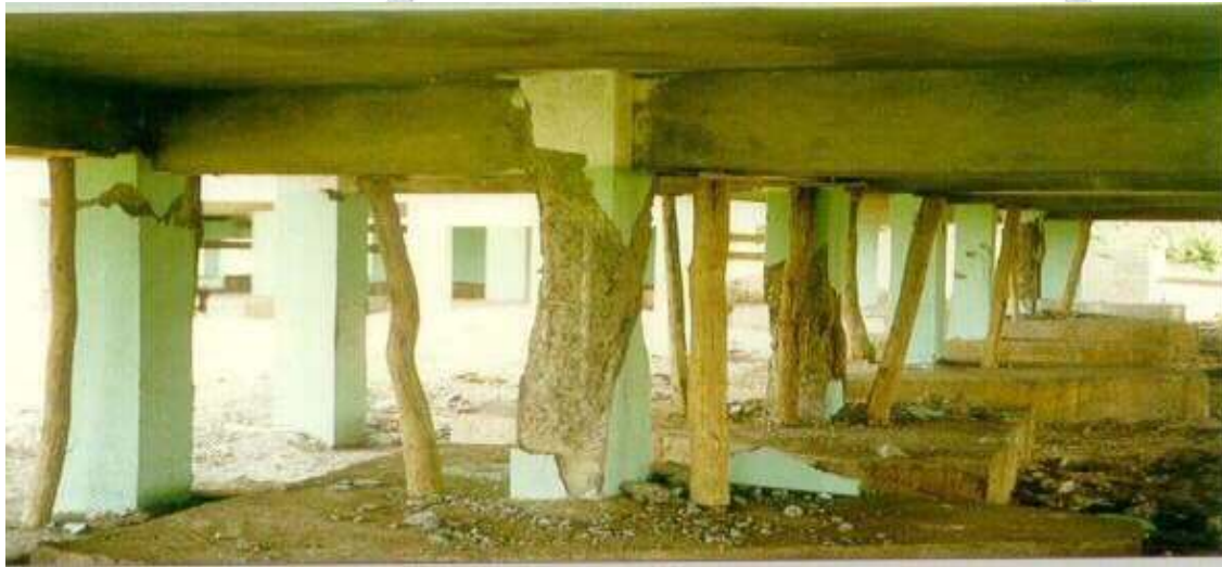
Figure 2 :: Damage to columns in the soft storey
