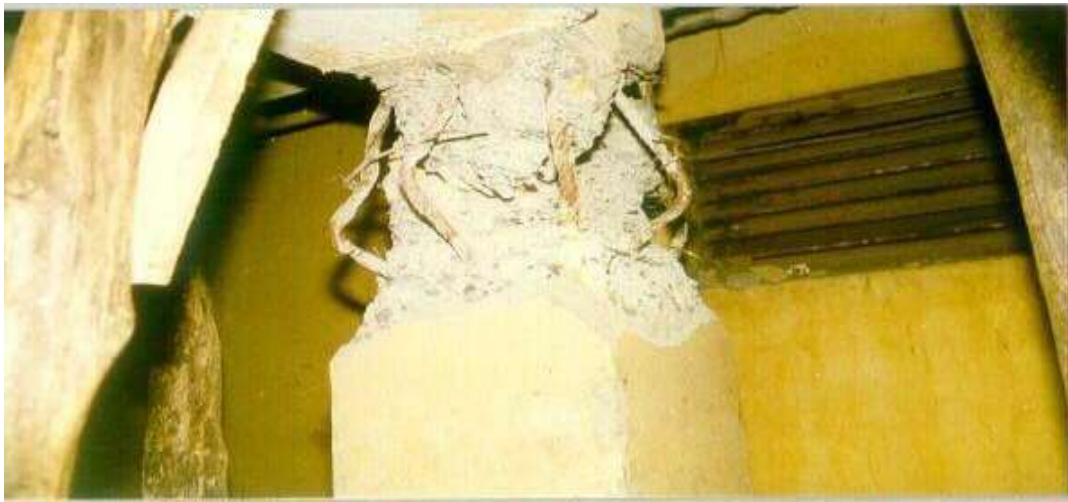
Figure 1 :: Damage to columns
