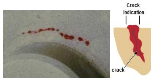
Fig 5.2 Visible Of Cracks
