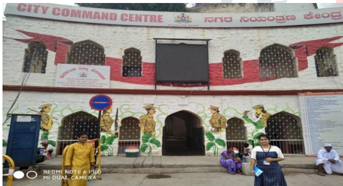
Figure: City Command Center, Kalaburagi.
