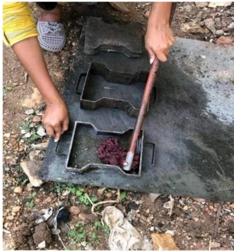
Fig: 4.4.3.Moulding of plastic sand mix
