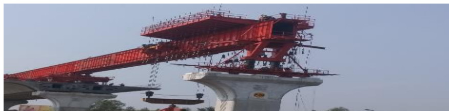
Fig.12 Box Girder Launching Gantry
