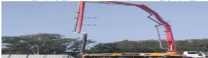
Fig.11 Boom Truck (Crane pouring concrete)
