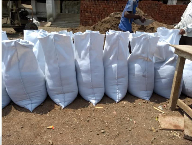
Geobags filled with sand ready for sewing
