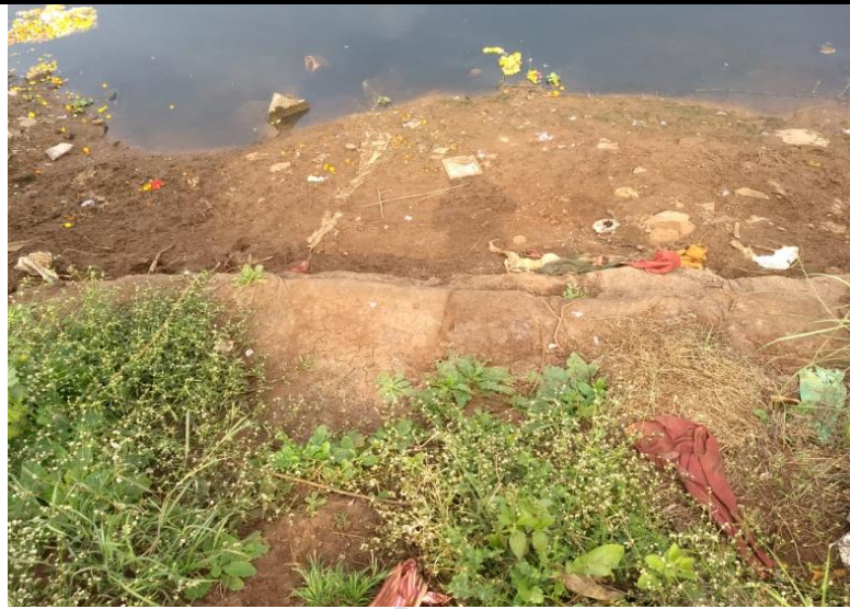
Vegetation growth on geobag installed sites indicating natural restoration of the bank to relative stability
