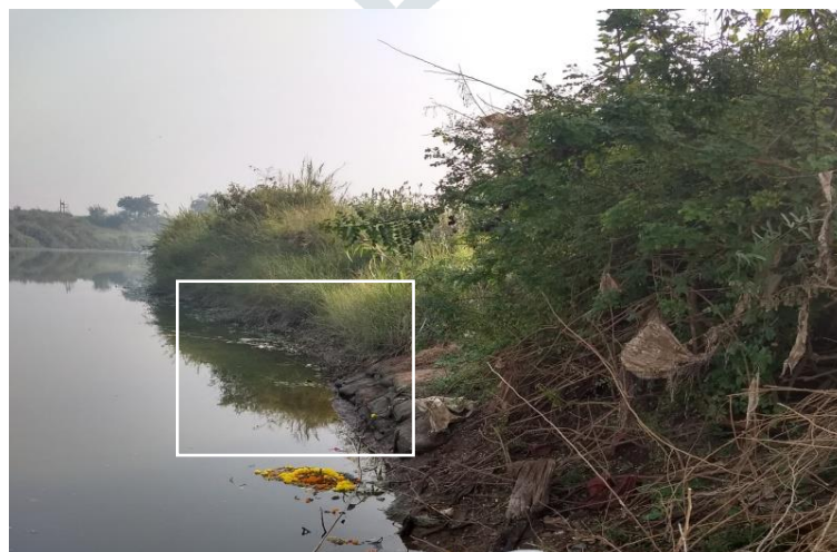
Retention of river bank due to installed geobags (post monsoon) preventing dislodging
