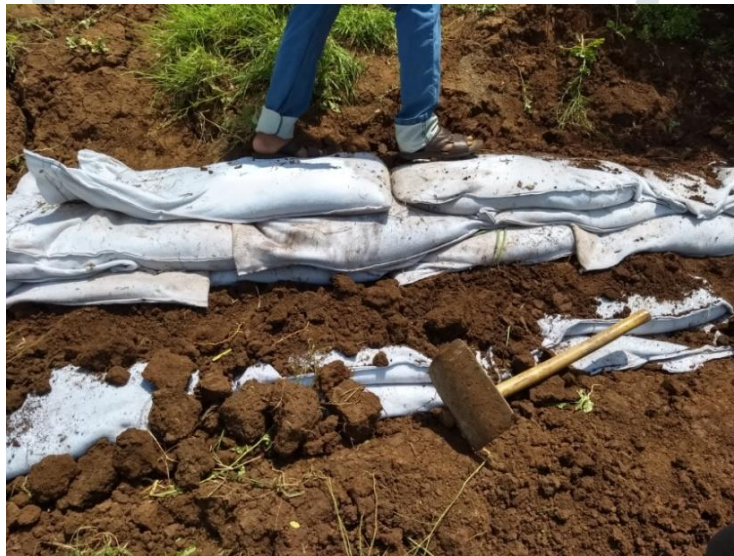
Laying of geobags on river bank site
