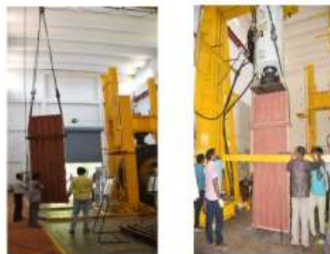
Fig 4. Lifting and positioning of SFCC wall panel
