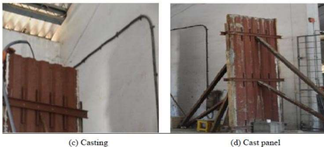
Fig 3. Casting of SFCC wall panel
