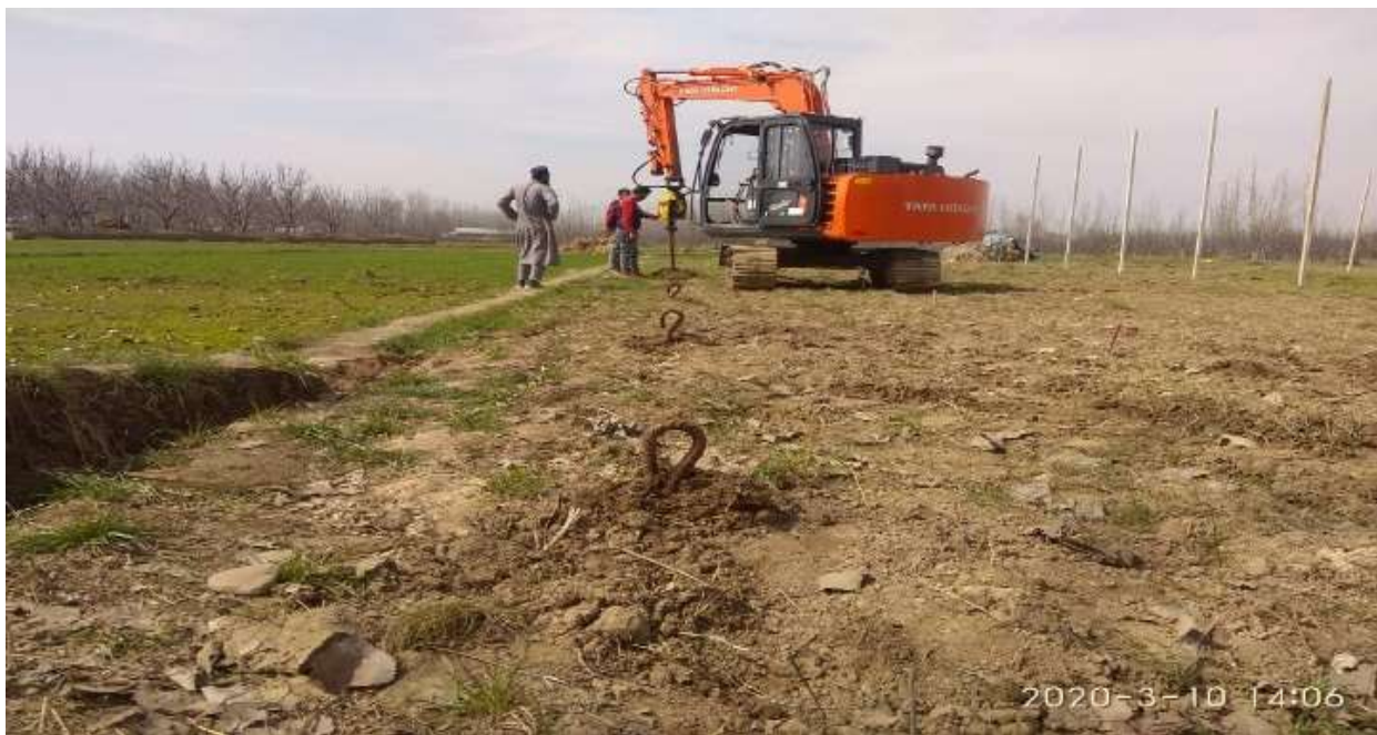
Figure 3. Installation of Anchorages at Pulwama J&K.
