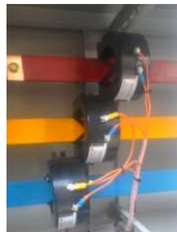
Figure4.Current Transformer
