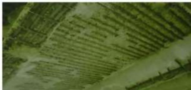
Figure 1:Correded reinforcing steel in concrete deck
