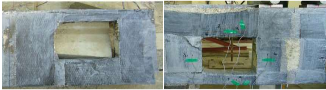
Fig-1 Carbon wrapping to the external surface near opening
