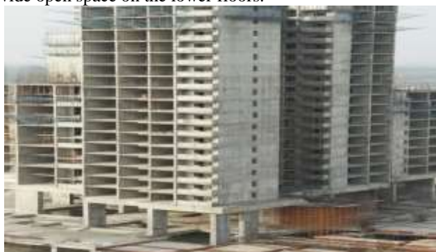
Figure 1:- Transfer slab With Shear wall
