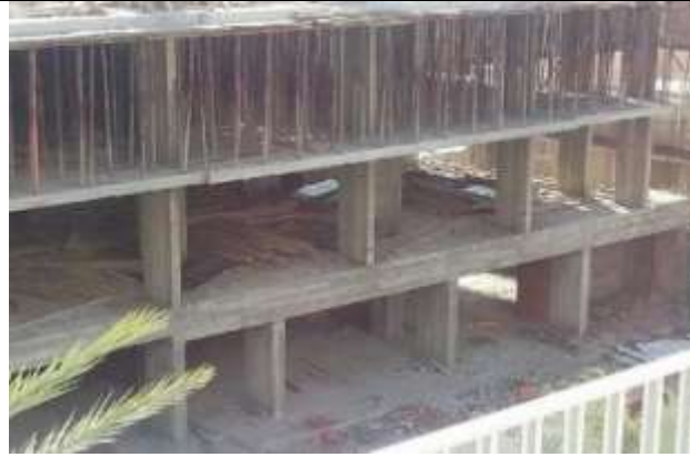
Figure 2:- Transfer slab With Column
