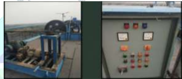
Image 1.1 Floodgate Mechanism
