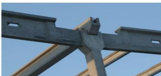
Fig1.1: Connection detail of post-tensioned precast specimen
