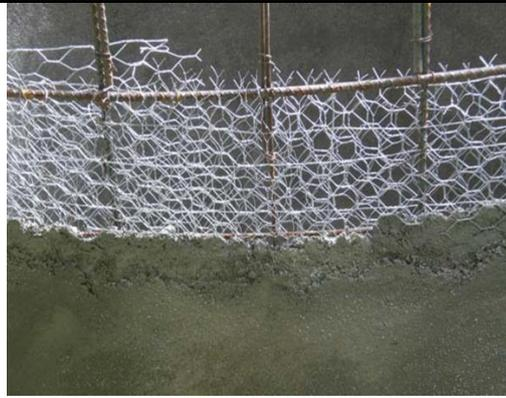
**Figure 1 Typical cross section of ferrocement structure**
