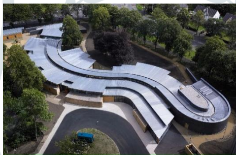
Figure 3: Hazelwood School Glasgow
