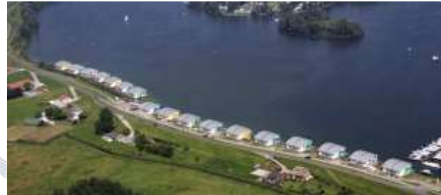
Figure 2. Floating and amphibious houses with access road and floating pier. Source: studio van hesse
