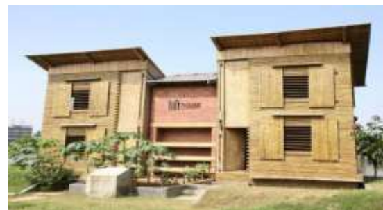
Figure3. Exterior bamboo treatment of lift house
