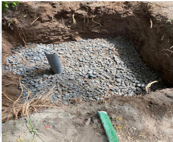
Figure 8 Material Filling Layers in Pit
