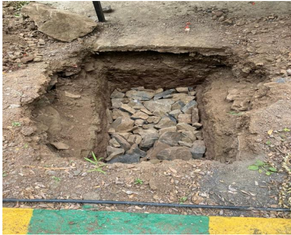
Figure 7 Material Filling in Pit
